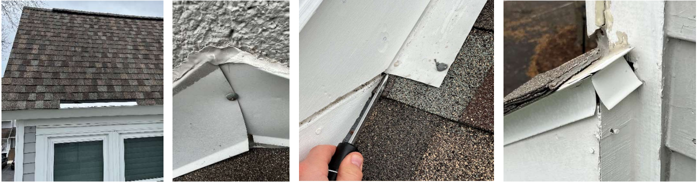
Photos 12, 13, 14, & 15 – Missing shingle at east gable roof (Left), Unsealed counter-flashing at ridge of chimney roof cricket (Center Left), Gap at roof end wall flashing and trim (Center Right), and Gaps at roof trim (Right).
