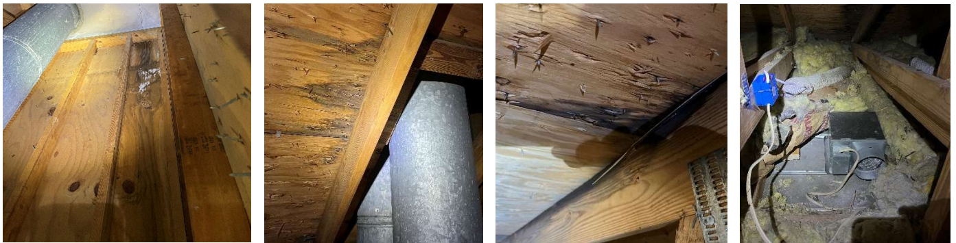
Photos 28, 29, 30, & 31 (Unit 205) – Damaged plywood sheathing at top of chimney interior (Left), Evidence of water infiltration/staining on roof decking (Center Left & Center Right), and Exhaust fan venting directly to attic space (Right).
