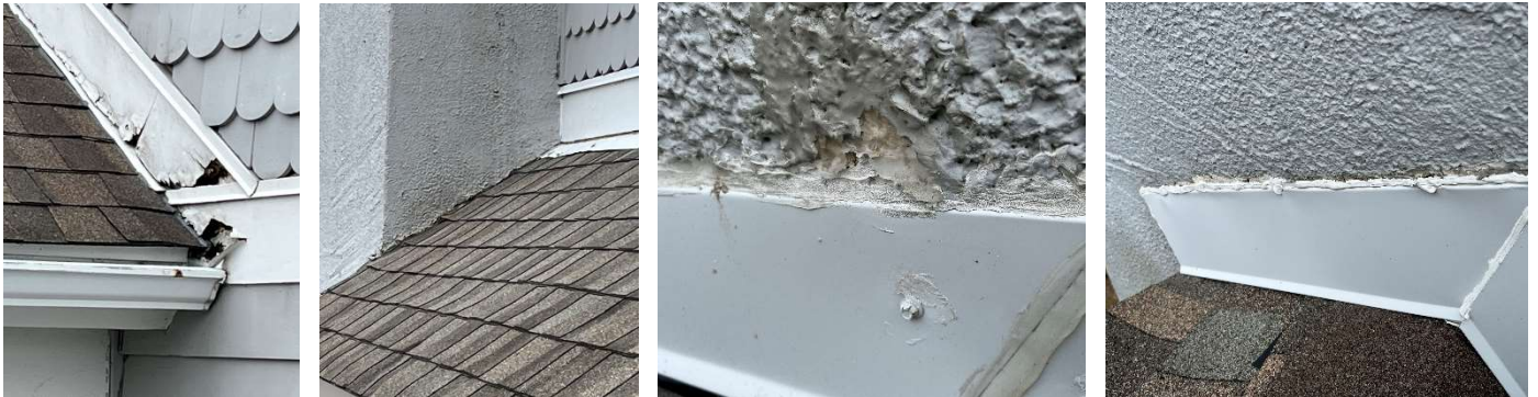
Photos 4, 5, 6, & 7 – Missing kick-out flashing (Left & Center Left), Degraded counterflashing sealant and tabby stucco coating at base of chimneys (Center Right & Right).
