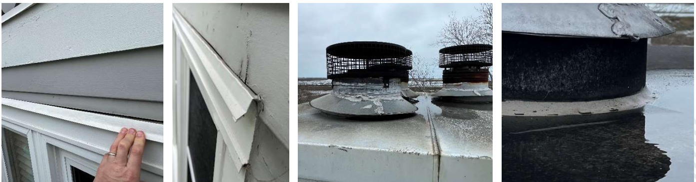
Photos 8, 9, 10, & 11 – Typical window trim flashing negatively sloped (Left & Center Left), Typical ponding water at chimney caps (Center Right), and Gaps at chimney cap/flue flange tabs (Right).
