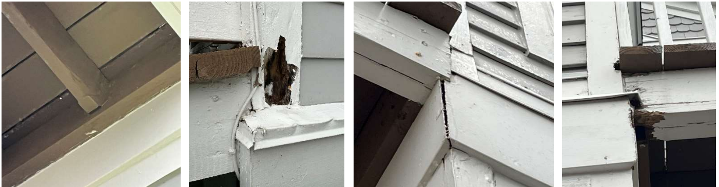
Photos 28, 29, 30, & 31 – Typical missing ledger flashing at upper level decks (Left), Typical corner trim rot (Center Left), Typical gap at corner trim (Center Right), and Typical rot damage to deck rim joist (Right).
