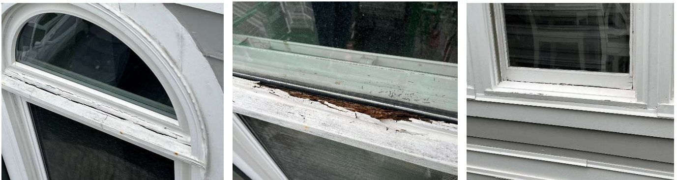
Photos 16, 17, & 18 – Rotted transom window sill (Left & Center), and Cracks, openings, and sealant delamination at window frames and trim (Right).
