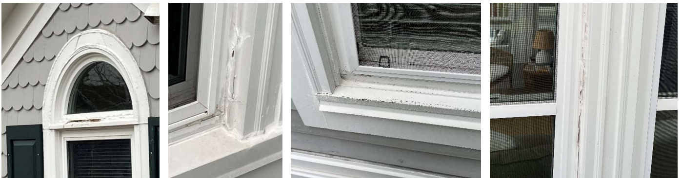
Photos 16, 17, 18, & 19 – Rotted transom window sill (Left), Cracks, openings, and sealant delamination at window frames and trim (Center Left, Center Right, & Right).
