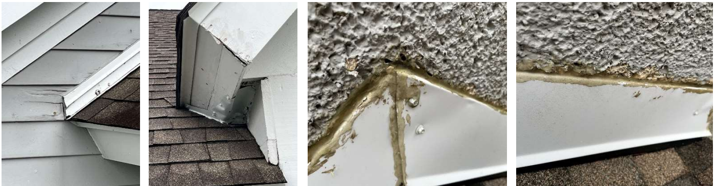
Photos 4, 5, 6, & 7 – Missing kick-out flashing (Left), Negatively sloped and sealed fascia trim repair (sheet metal) (Center Left), Degraded counterflashing sealant and tabby stucco coating at base of chimneys (Center Right & Right).
