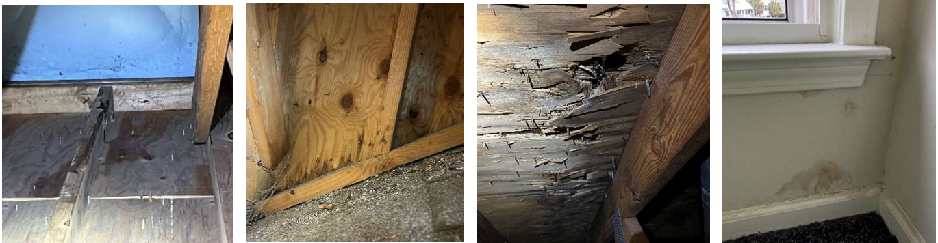
Photos 27, 28, 29, & 30 (Unit 306) – Damaged plywood sheathing at top of chimney interior (Left), Evidence of water infiltration/staining on roof decking (Center Left), Damage to roof decking at base of chimney (Center Right), and Evidence of water infiltration/staining on interior finishes below windows (Right).
