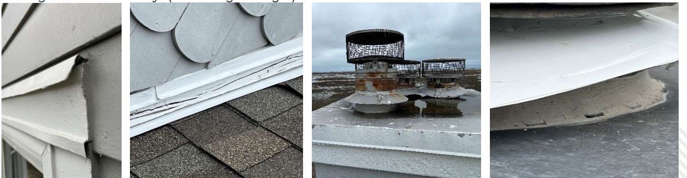
Photos 8, 9, 10, & 11 – Typical window trim flashing negatively sloped (Left), Typical end wall trim cracked & damaged (Center Left), Typical ponding water at chimney caps (Center Right), and Gaps at chimney cap/flue flange tabs (Right).
