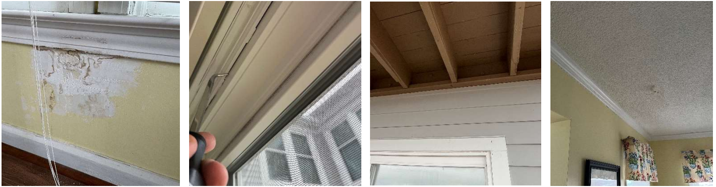
Photos 24, 25, 26, & 27 (Unit 202) – Damaged interior wall finishes (Left), Reported location of water intrusion at window frame interior (Center Left), Typical missing ledger flashing (Center Right), and Interior ceiling damage adjacent to exterior deck (Right).
