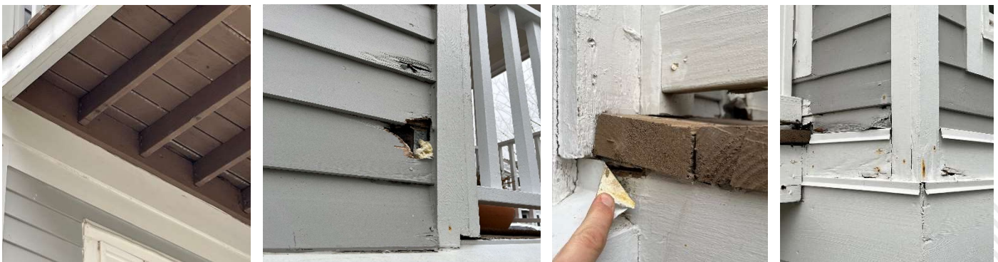
Photos 19, 20, 21, & 22 – Typical missing ledger flashing at upper level decks (Left), Typical siding rot (Center Left), Untermated siding flashing at deck (Center Right), and Typical rot damage to siding & trim (Right).
