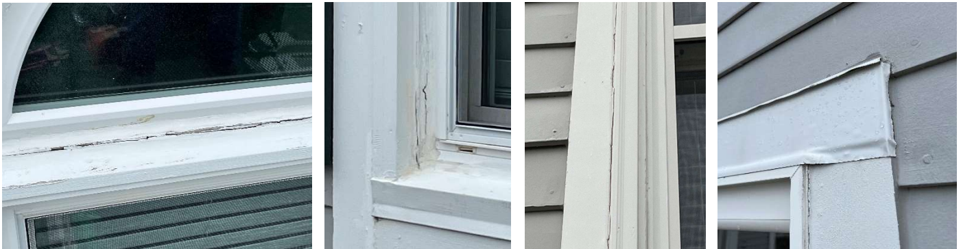
Photos 16, 17, 18, & 19 – Rotted transom window sill (Left), Cracks, openings, and sealant delamination at window frames and trim (Center Left & Center Right), and Evidence of prior temporary repairs to fenestration framing (Right).
