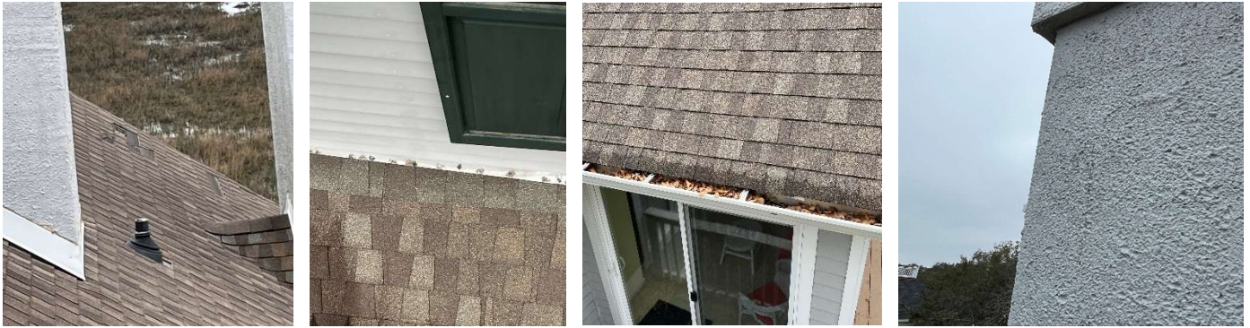
Photos 12, 13, 14, & 15 – Missing shingles at upper roof south elevation (Left), Missing shingles at low roof apron flashing (Center Left), Gutter debris (Center Right), and Typical cracking of tabby stucco at chimneys (Right).
