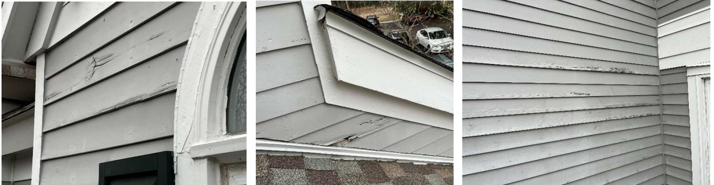
Photos 1, 2, & 3 – Typical rotted siding throughout, numerous locations, multiple building elevations and areas.
