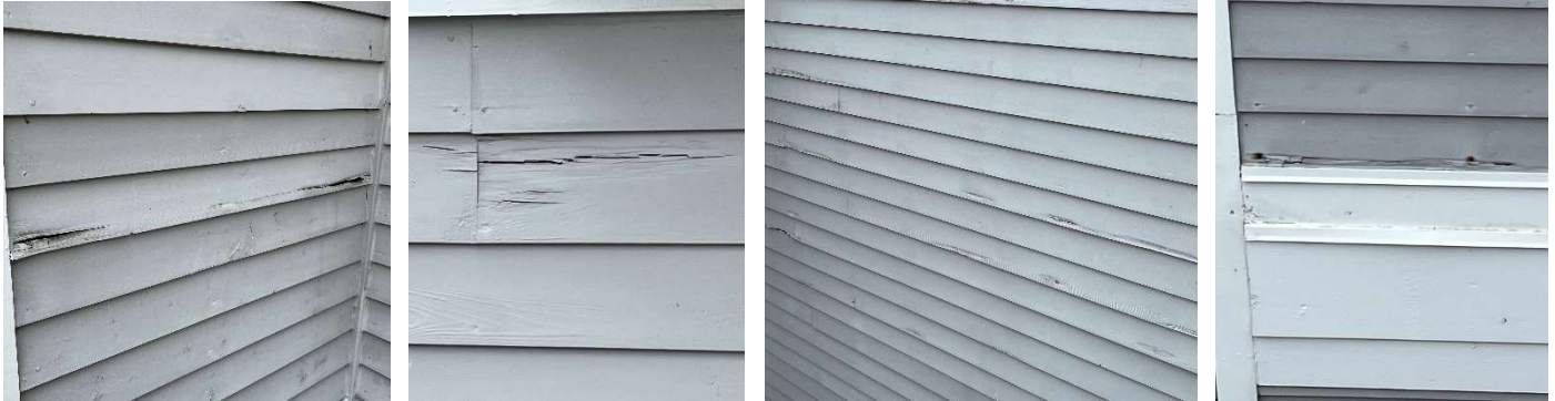
Photos 1, 2, 3, & 4 – Typical rotted siding throughout, numerous locations, multiple building elevations and areas.
