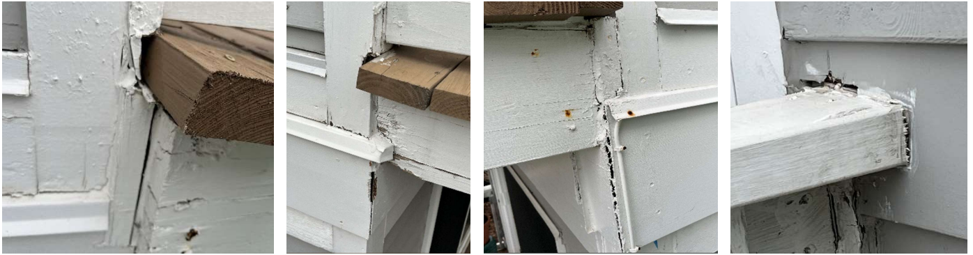
Photos 24, 25, 26, & 27 – Typical gaps, openings, and missing flashing at upper level decks and trim.
