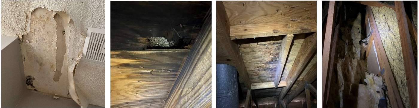
Photos 23, 24, 25, & 26 (Unit 305) – Damaged interior ceiling finishes (Left), Damaged plywood roof decking at base of chimney (Center Left), Evidence of water infiltration/staining on roof decking (Center Right), and Typical missing attic insulation at clerestory walls (Right).
