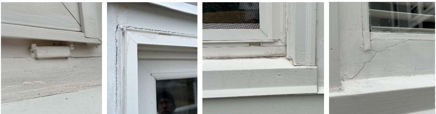
Photos 20, 21, 22, & 23 – Window sill weep painted closed (Left), Cracks, openings, and sealant delamination at window frames and trim (Center Left, Center Right, & Right).
