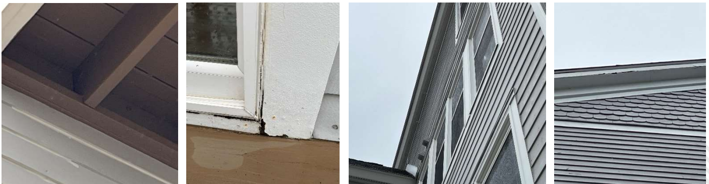
Photos 20, 21, 22, & 23 – Typical missing ledger flashing at upper level decks (Left), Typical trim rot at slider trim in contact with decking (Center Left), Bowed clapboards at east elevation (Center Right), and Typical rot damage to roof rake (Right).
