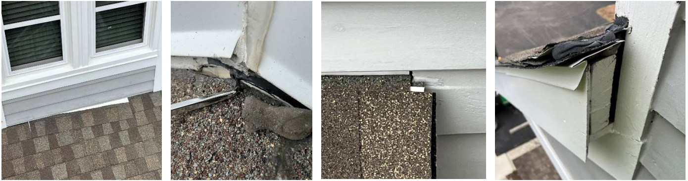
Photos 12, 13, 14, & 15 – Detached shingle at low roof west elevation (Left), Unsealed counter-flashing at ridge of chimney roof cricket (Center Left), Gap at end of roof apron wall flashing (Center Right), and Gaps at roof trim (Right).
