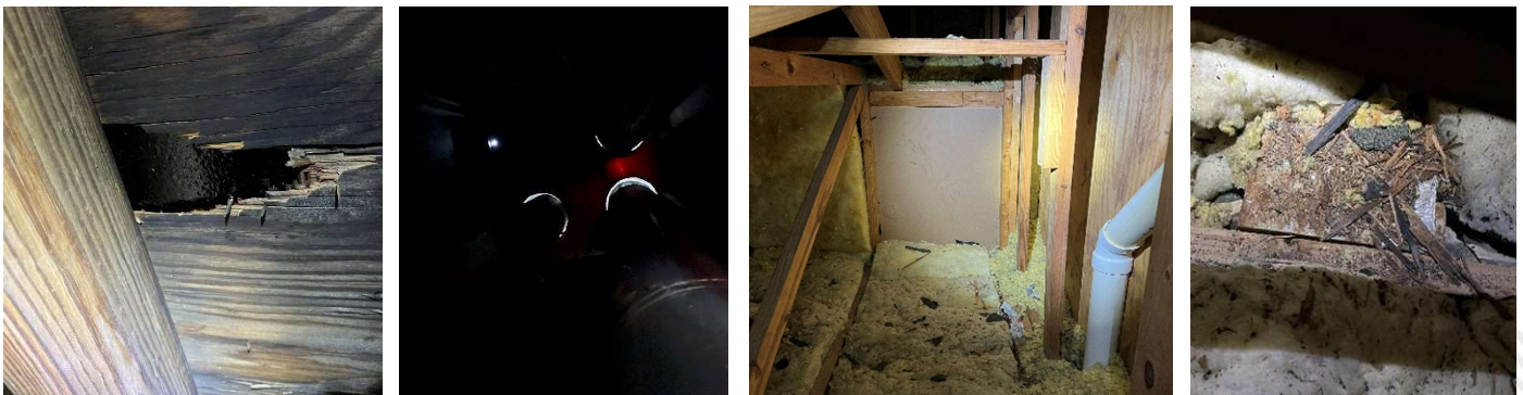
Photos 31, 32, 33, & 34 (Unit 108) – Damaged plywood roof decking at base of chimney (Left), Pinhole (upper left) in chimney cap (Center Left), Typical missing attic insulation at clerestory walls (Center Right), and Exhaust fan venting directly to attic space (Right).
