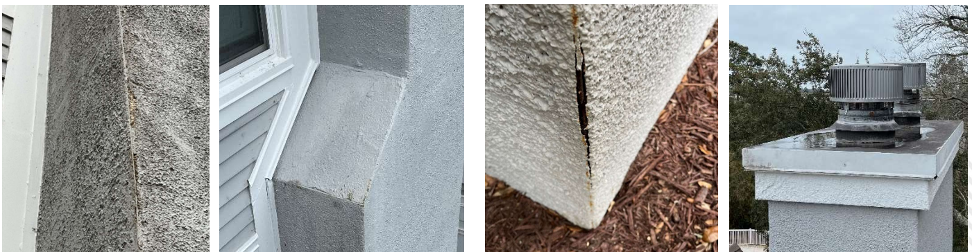
Photos 8, 9, 10, & 11 – Typical edge corrosion and decomposition of chimney tabby stucco (Left, Center Left, & Center Right), and Typical ponding water at chimney caps (Right).
